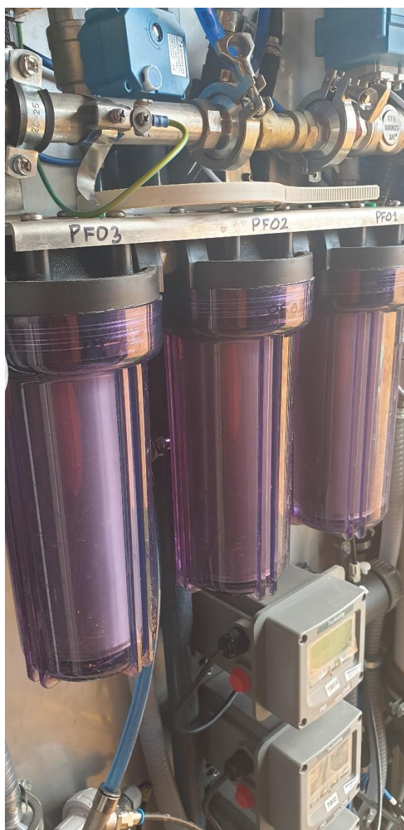
Figure 11 Pre-filtration/particulate filtration housing (photo credit: Trevor Harvey).
